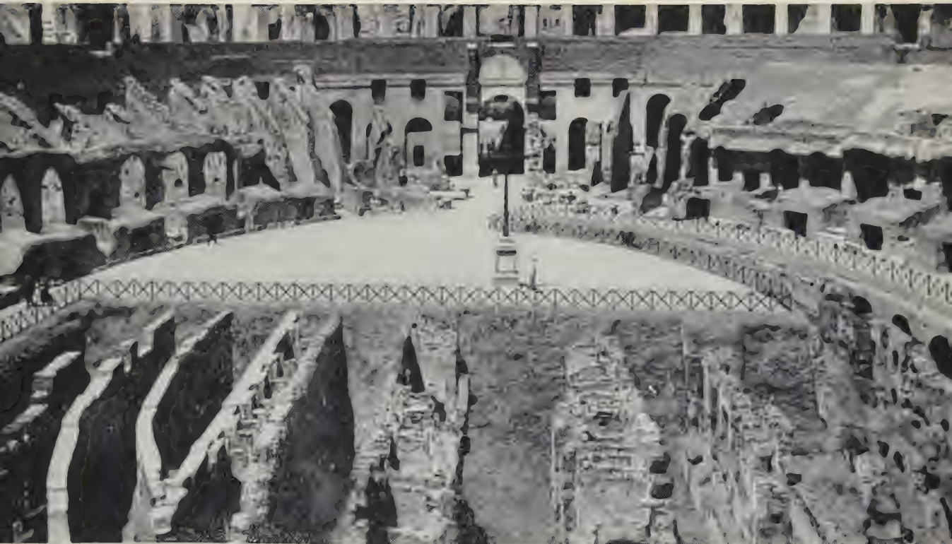
Most of the floor of the Colosseum has been removed, to show the substructure
